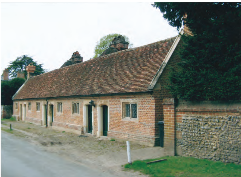
Fig. 13.4 Terrace of almshouses, brick with stone dressings, Mapledurham
